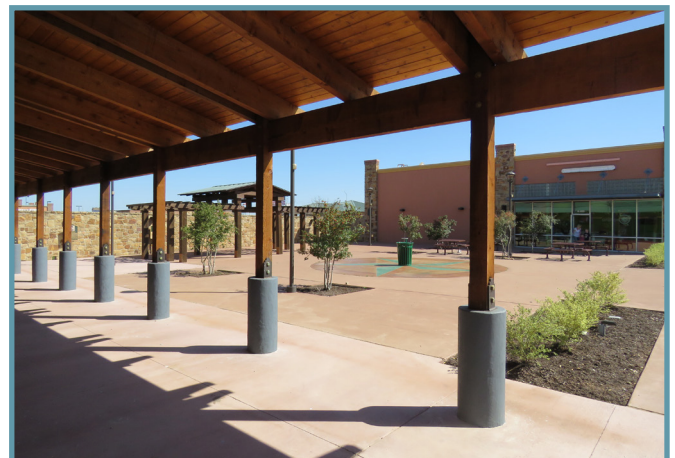
Typically associated with residential development, many communities are now requiring common areas, public gathering spaces, and recreational amenities as part of non-residential development (above).
